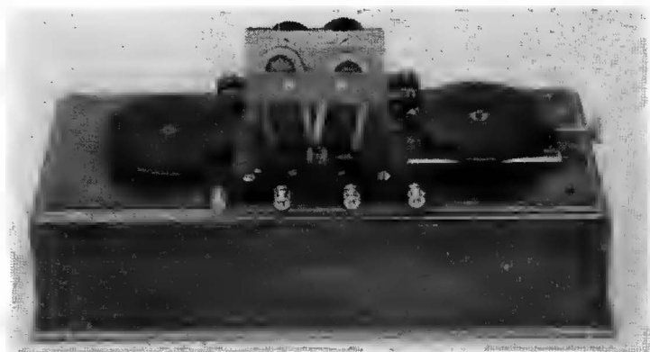
Fig 5.21 Marconi's moving-band hysteresis detector [Science Museum Photograph]
