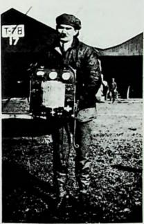
Fig. 7-7. Early type of aircraft radiophone transmitter, held by Lee de Forest.
