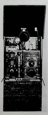
Fig. 12-26. Telefunken transmitter, made in 1915, using EVN129 tube. (Reproduced from Zenneck and Rukop, (Lehrbuch der drahtlose Telegraphie.)
