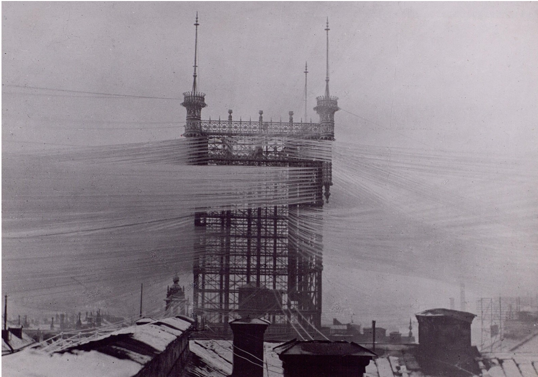
Stockholm Central Telephone/Telegraph Tower
